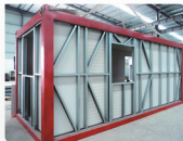
4. 硅钙板安装 CALCIUM SILICATE BOARD INSTALLATION
