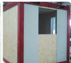
5. 外墙水泥纤维板安装 EXTERIOR WALL CEMENT FIBERBOARD INSTALLATION
